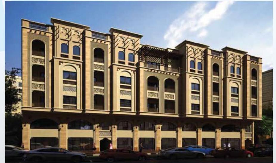
B + G + M + 3 TYP + ROOF, PLOT NO. 312-2377 @ AL SOUQ AL KABEER, DUBAI.
