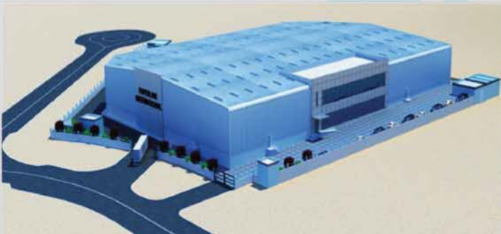
PAPERLINK INTERNATIONAL-WAREHOUSE & OFFICE, PLOT NO. S20108 @ JAFZA, DUBAI
