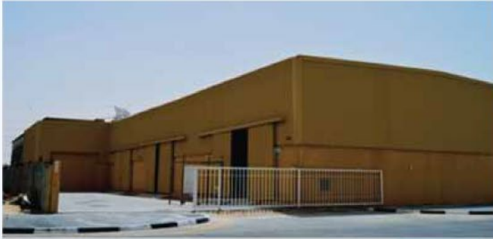
GROUND FLOOR WAREHOUSE @RAS AL KHOR, DUBAI
